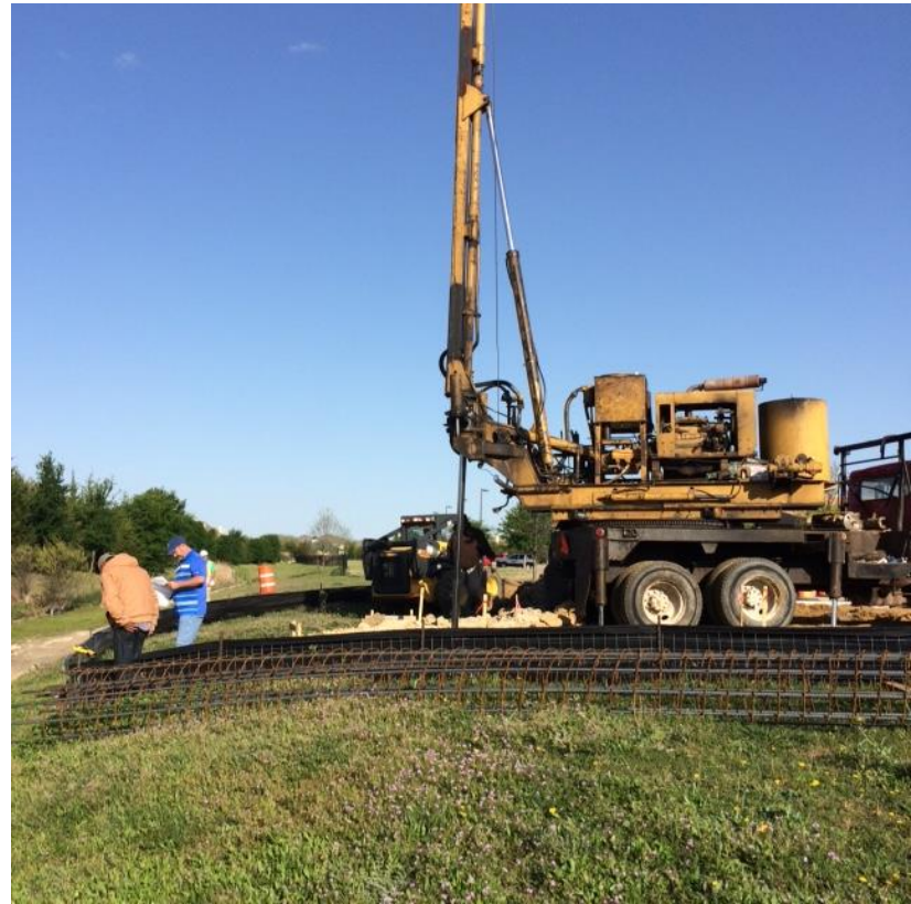
Drilling for bridge piers
