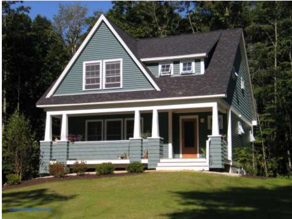
Colonial Revival Twist Style Architectural Example
