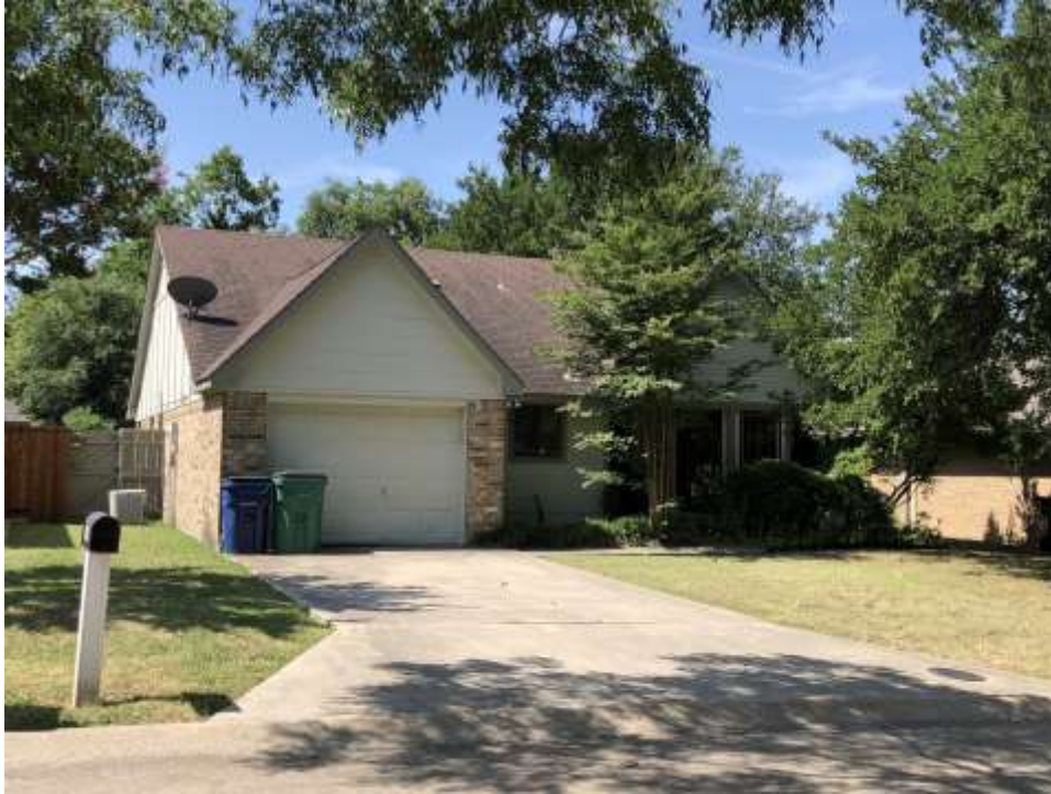
108 East Graham Street (Immediately Across Graham Street facing Development) Style: Traditional (Illustrates existing character, not Developer's proposed character)
