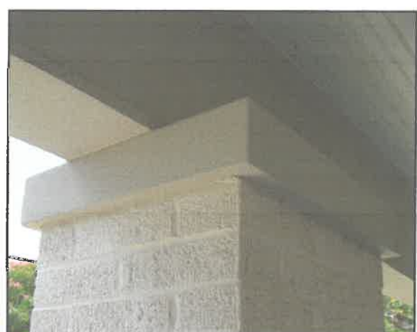
Plain limestone cap on brick column
