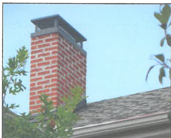
Chimney made of "carpet" brick
