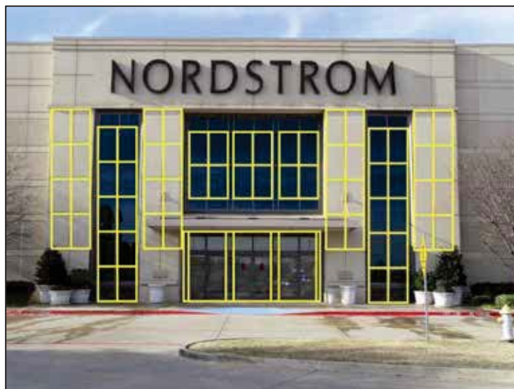
Figure 4.09.03.2: Example of Windows and Entrances Designed with Concepts from the Golden Mean and Fibonacci Sequence
