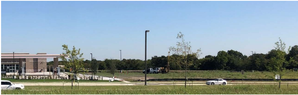
Looking Southeast from across Hardin
