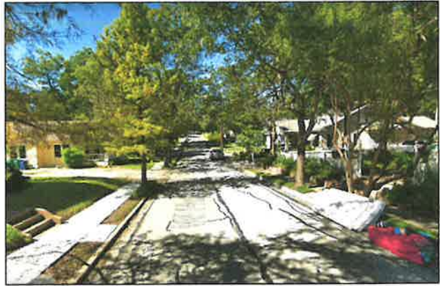
View looking West on W. Hunt Street
