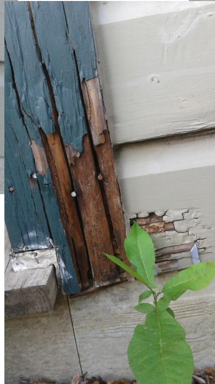
Wood rot & peeling paint from sprinkler head design
