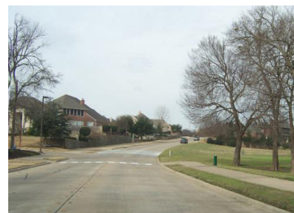
Collector street in McKinney
