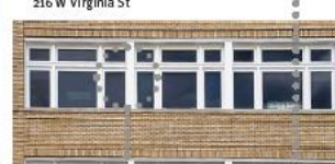
GROUPED WINDOWS 208 E Louisiana St
