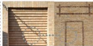
INSET BRICK PANELS 107 1/2 E Virginia Parkway
