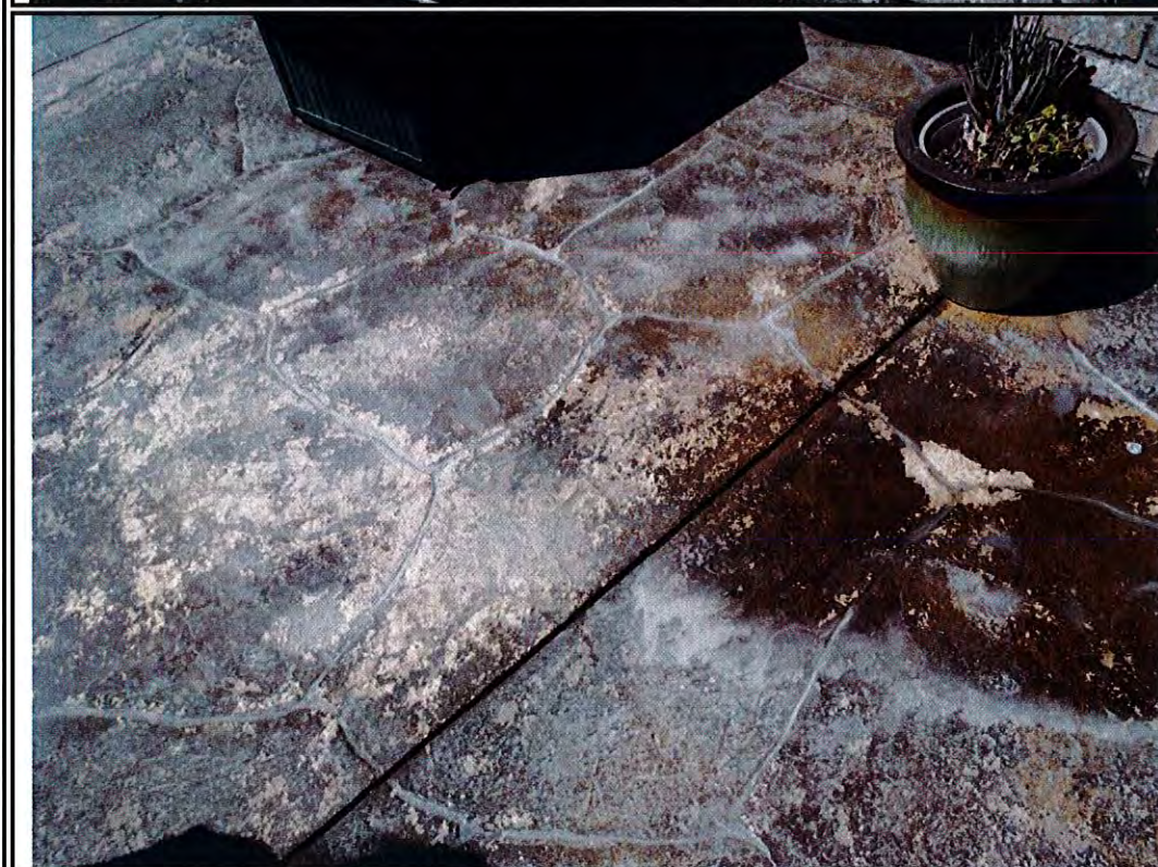
Photograph #2 Date: 7/19/19 Time: 11:00 am Comments: Photo showing the impact of emitted dust. Cement is discoloring the property. Clean patch shown on right side.
