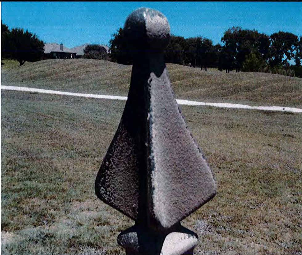
Photograph #6 Date: 7/19/19 Time: 11:00 am Comments: Photo showing extent of impact of emissions event. Cement adheres to fencing in an opaque layer. Grass is discolored by cement dust.
