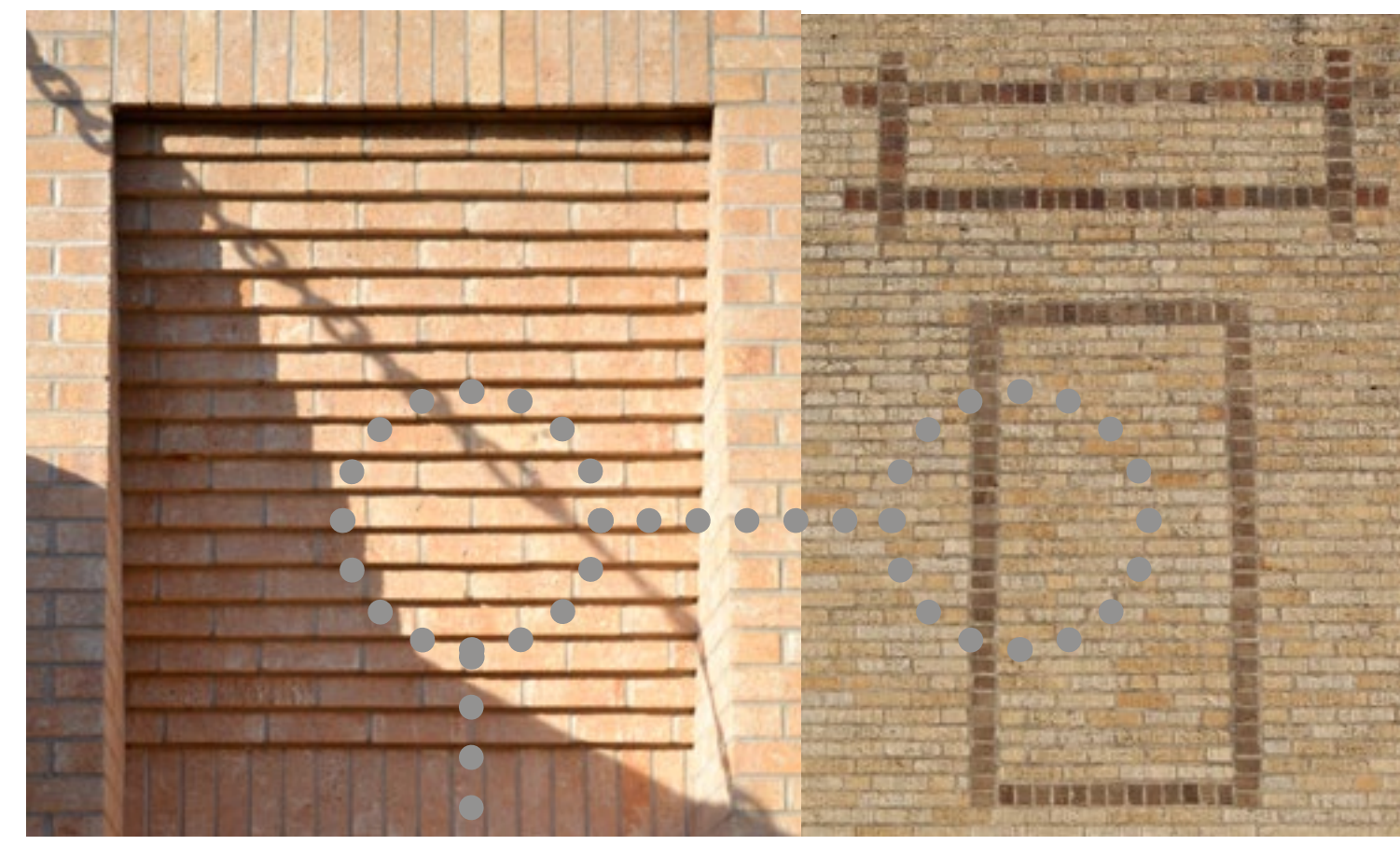
INSET BRICK PANELS 107 1/2 E. Virginia Parkway
