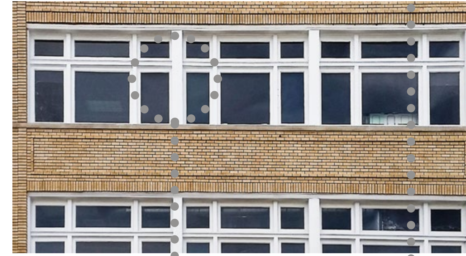
GROUPED WINDOWS 208 E Louisiana St
