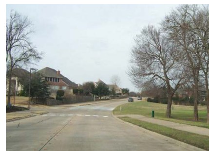
Collector street in McKinney
