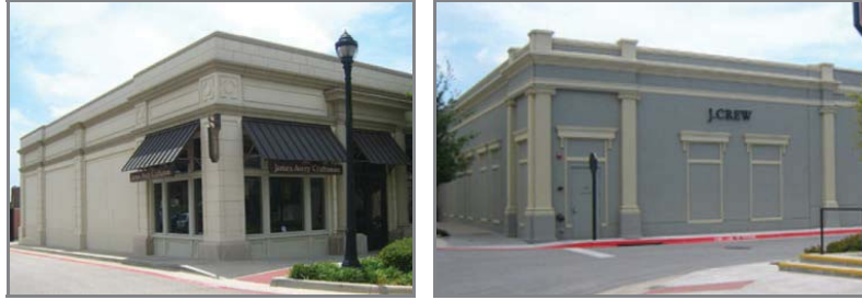
Images showing the side and rear façades buildings finished to match the color and materials of the front facades
