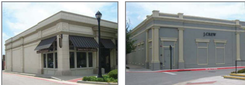
Images showing the side and rear façades buildings finished to match the color and materials of the front façades
