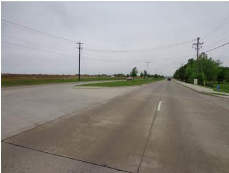
VIEW OF LAKE FOREST DRIVE FACING SOUTH
