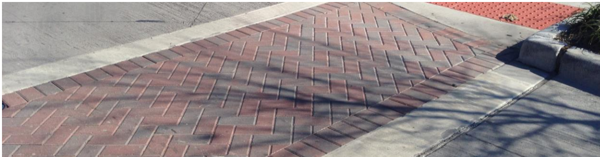
Crosswalk with Pavers
