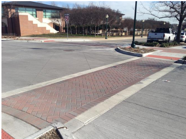
Crosswalk with Pavers
