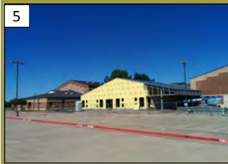
5 Johnson Elementary (MISD) 3400 Ash Ln. Valuation: $3.2 million Permit Issuance: January 2016
