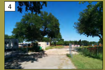
4 Samaritan Inn 1514 McDonald St. Valuation: $5.5 million Permit Issuance: January 2016
