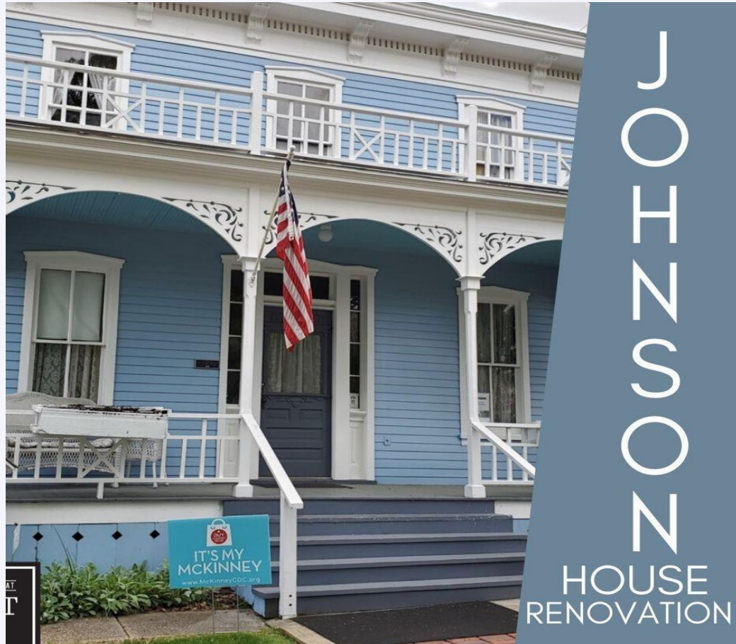
Renovations at Chestnut Square
