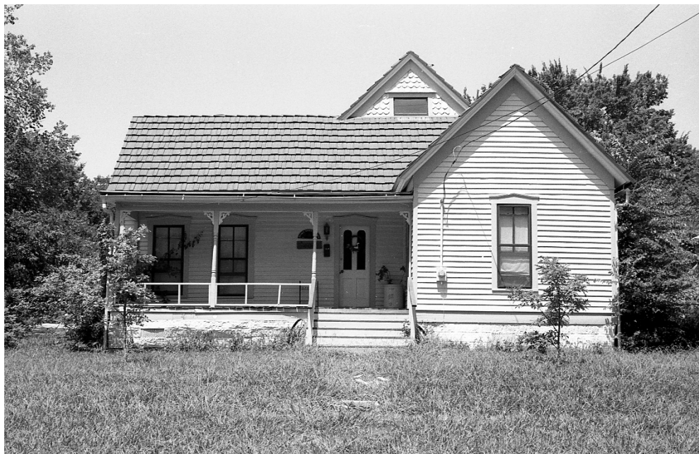
Front View- from the east
