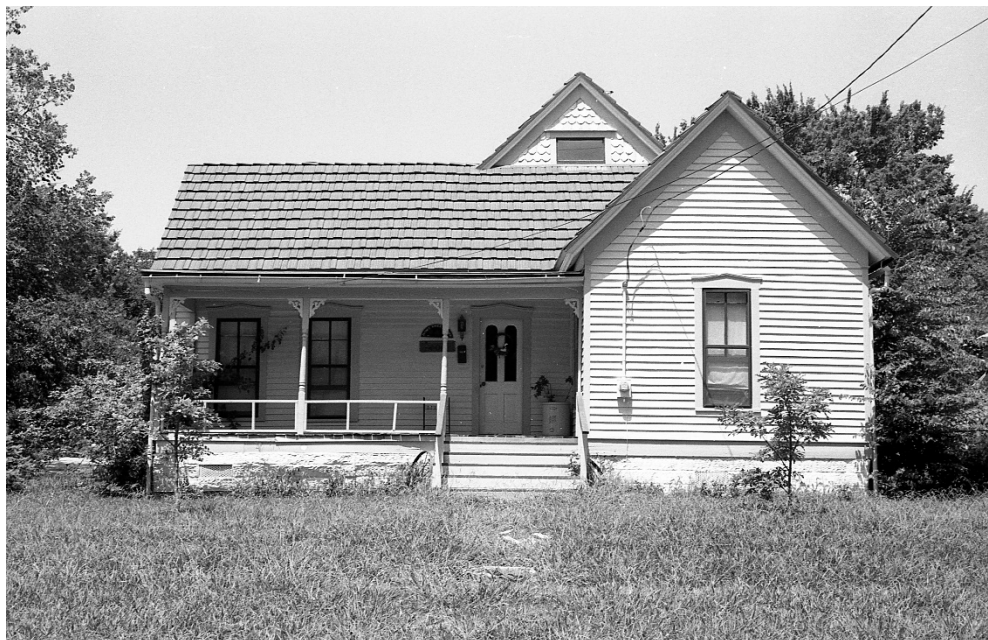
Front View- from the east
