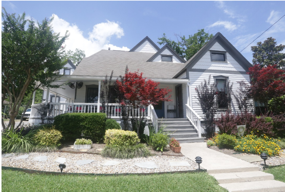
Front View- from the east
