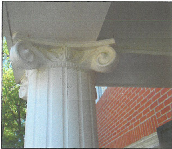
Ionic capitals that now decorate the portico columns were added after 1985. The original column appears to have been ornamented with a simple Tuscan base and capital.
