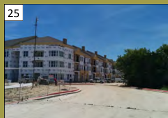
25 McKinney Urban Village 201 McKinney Village Pkwy. Valuation: $21 million Permit Issuance: January 2015
