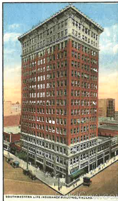
SOUTHWESTERN LIFE INSURANCE BUILDING, DALLAS, TEXAS
