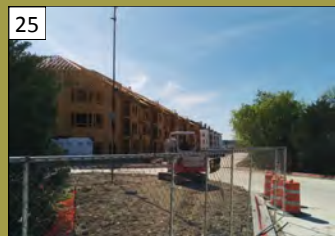
25 McKinney Urban Village 2500 S. McDonald St. Valuation: $21 million Permit Issuance: January 2015
