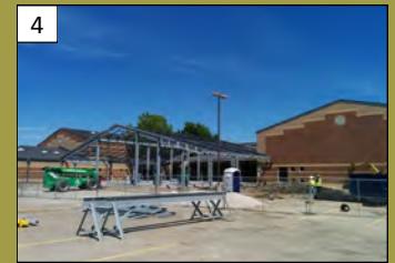
Johnson Elementary (MISD) 3400 Ash Ln. Valuation: $3.2 million Permit Issuance: January 2016
