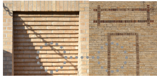
INSET BRICK PANELS 107 1/2 E. Virginia Parkway
