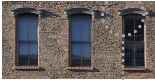
ARCHED WINDOW HEAD DETAILING 228 E Louisiana St
