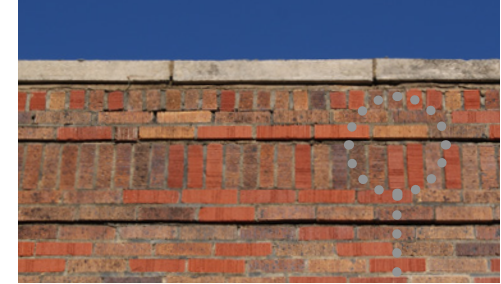
BRICK PARAPET DETAILING 214 N Kentucky St
