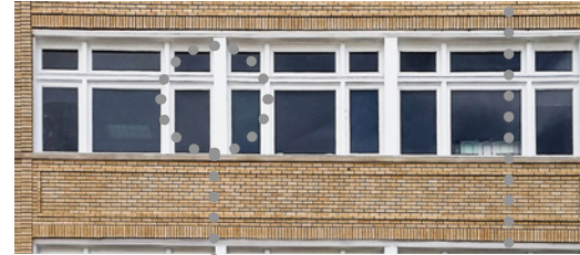
GROUPED WINDOWS 208 E Louisiana St
