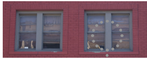
FRAMED WINDOWS INSET IN BRICK 107 W Louisiana St
