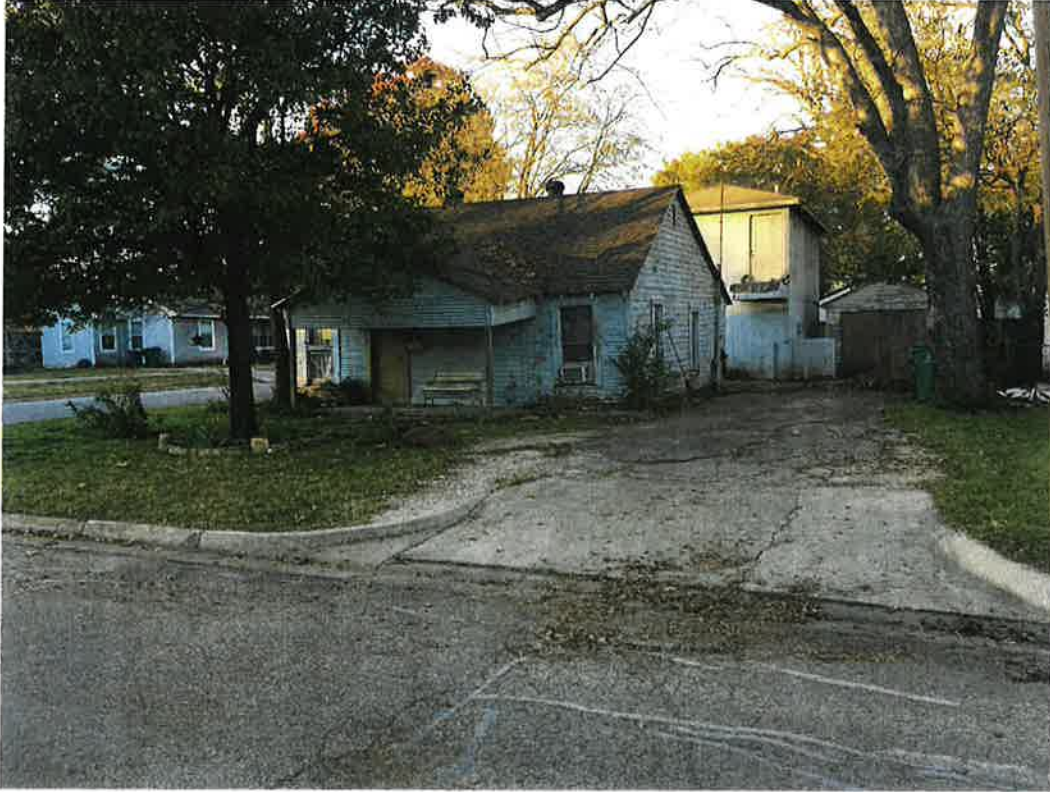
PHOTO 1 – South facing front of house with 2 story shop behind.
