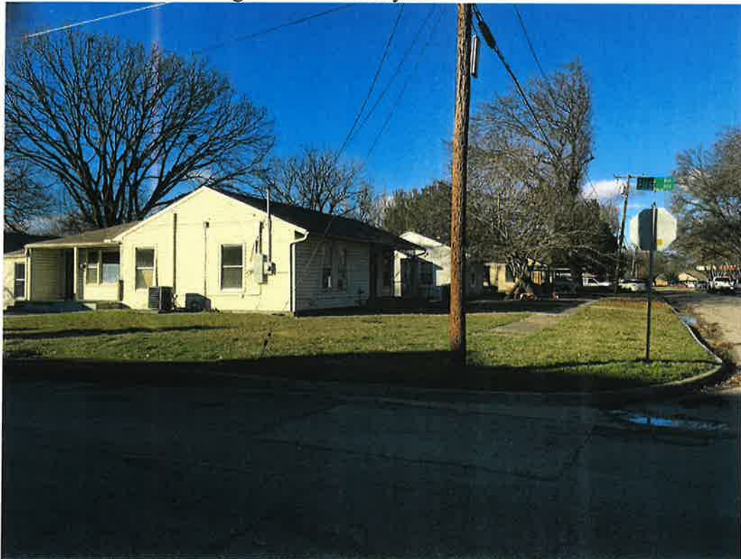
PHOTO 6 – Existing home on NW corner of Bradley and First.
