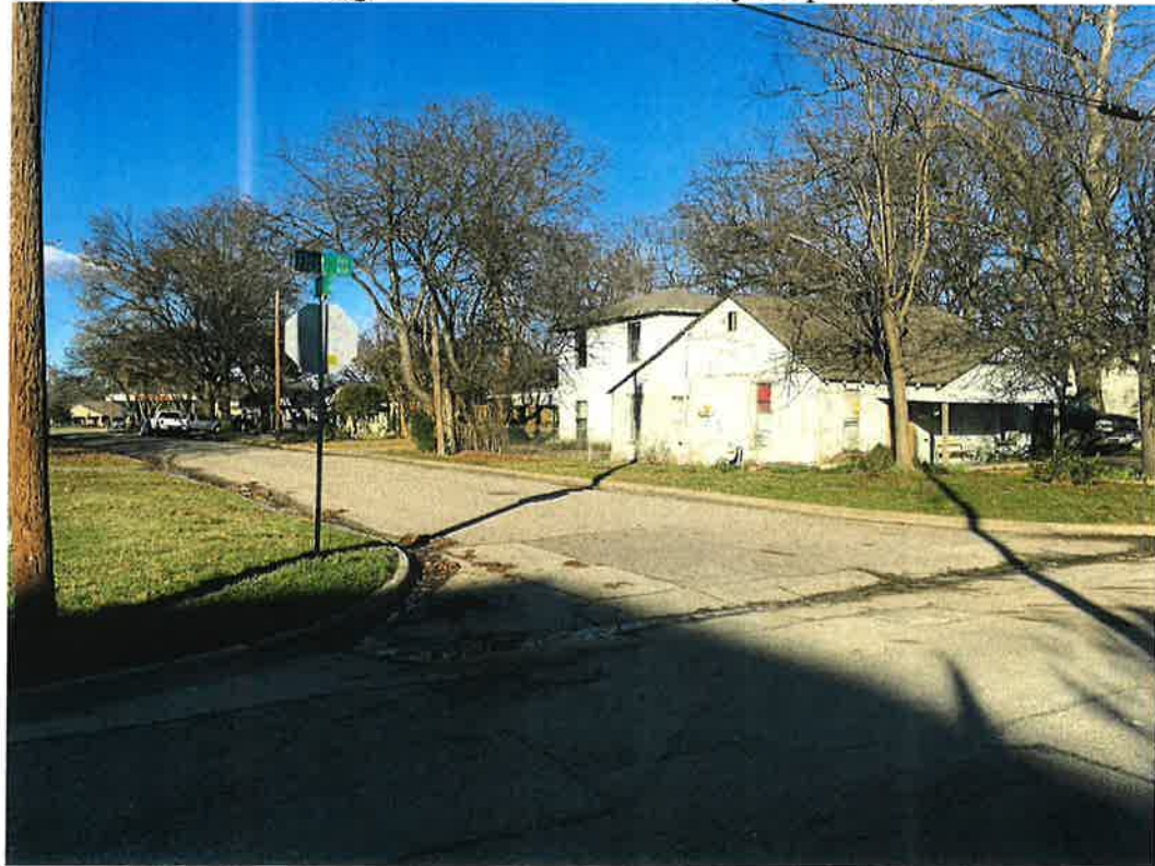
PHOTO 2 – West side of house facing Bradley Street.
