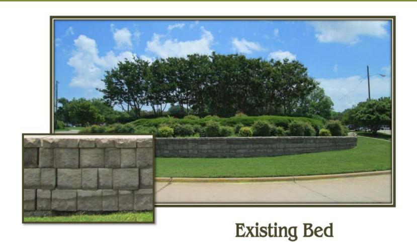
Wall is constructed of split faced concrete block.
