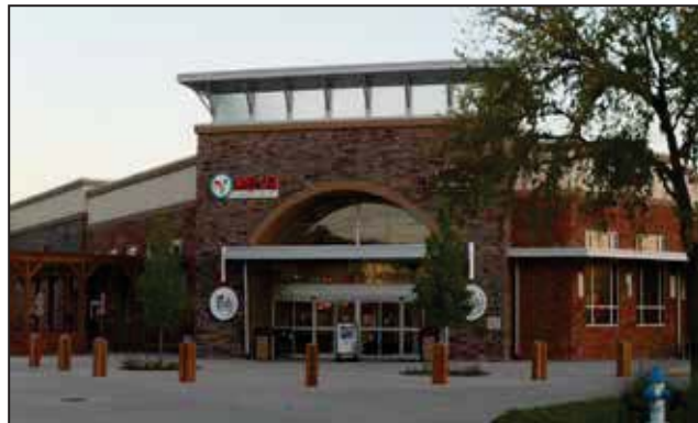
Figure 4.09.03.4: Building with Sheltered Entry
