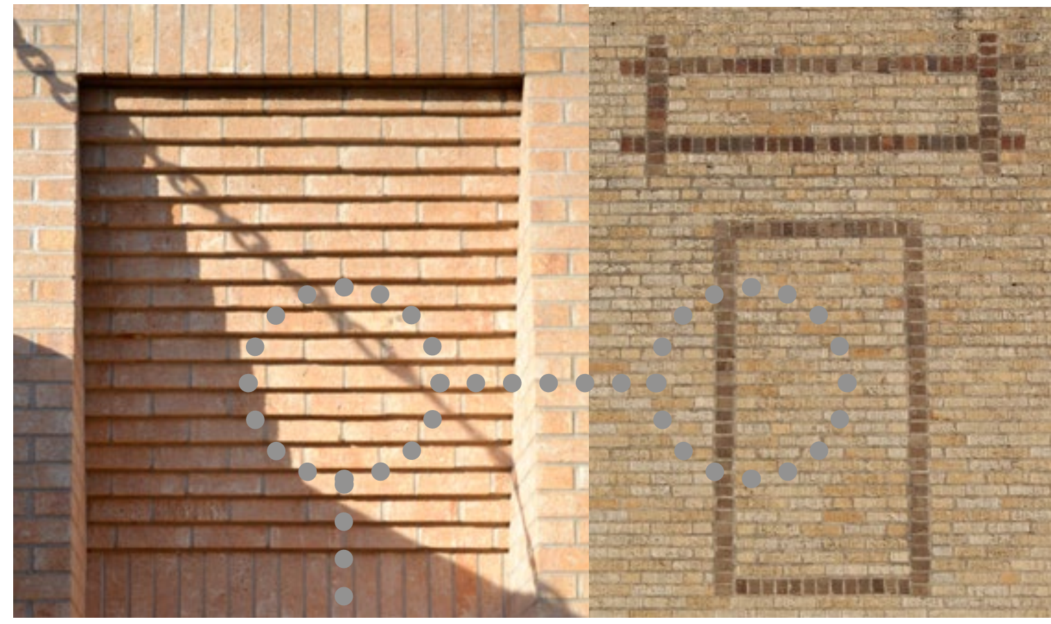
INSET BRICK PANELS 107 1/2 E. Virginia Parkway
