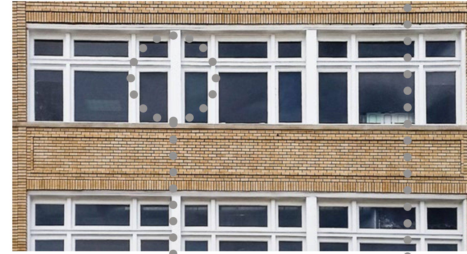
GROUPED WINDOWS 208 E Louisiana St
