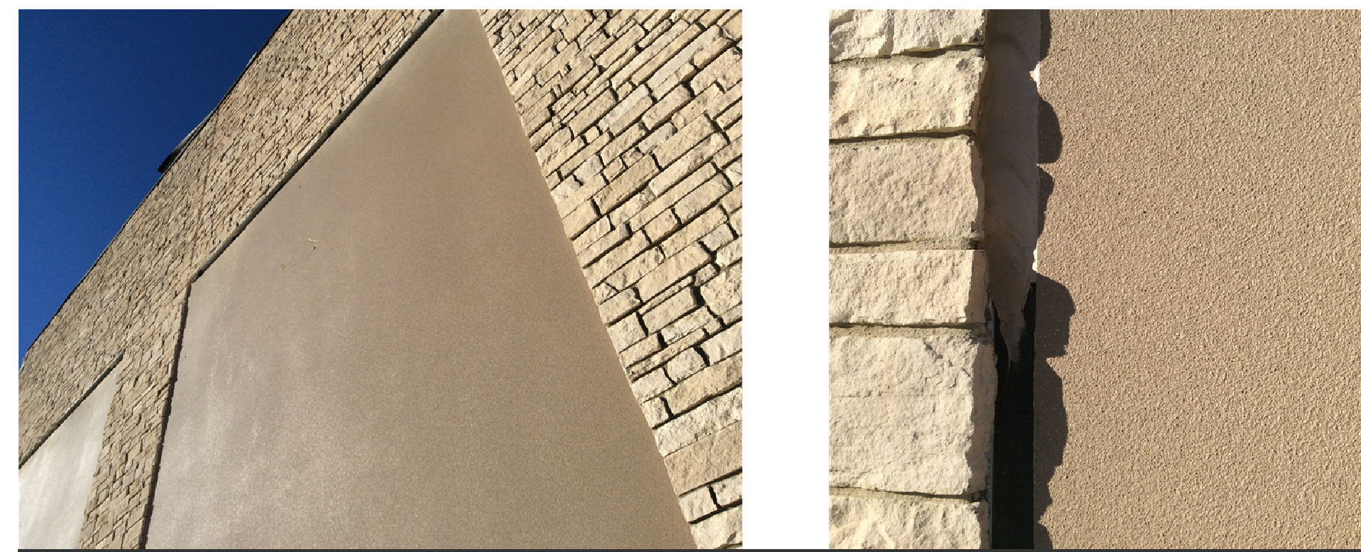
ARCHITECTURALLY FINISHED TILT WALL EXAMPLES
