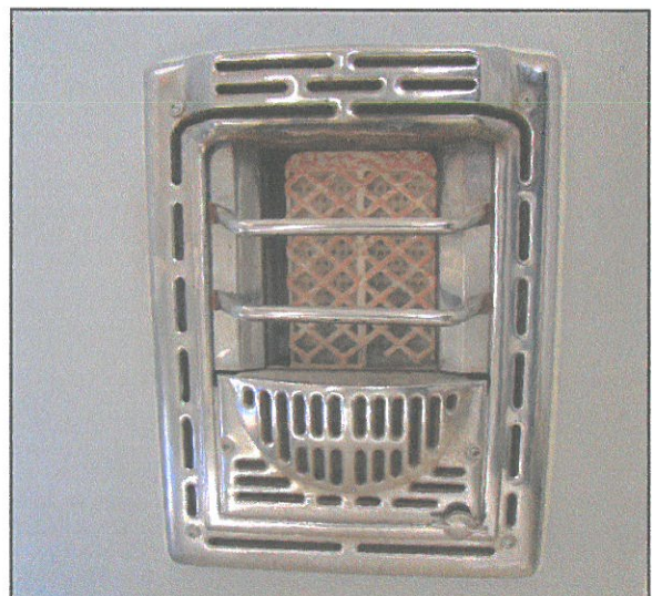
Chrome-plated bathroom gas-heater
