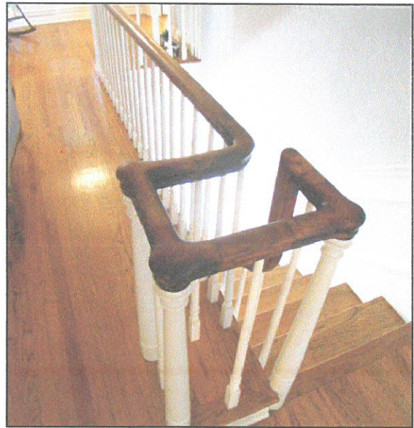
Banister railing detail
