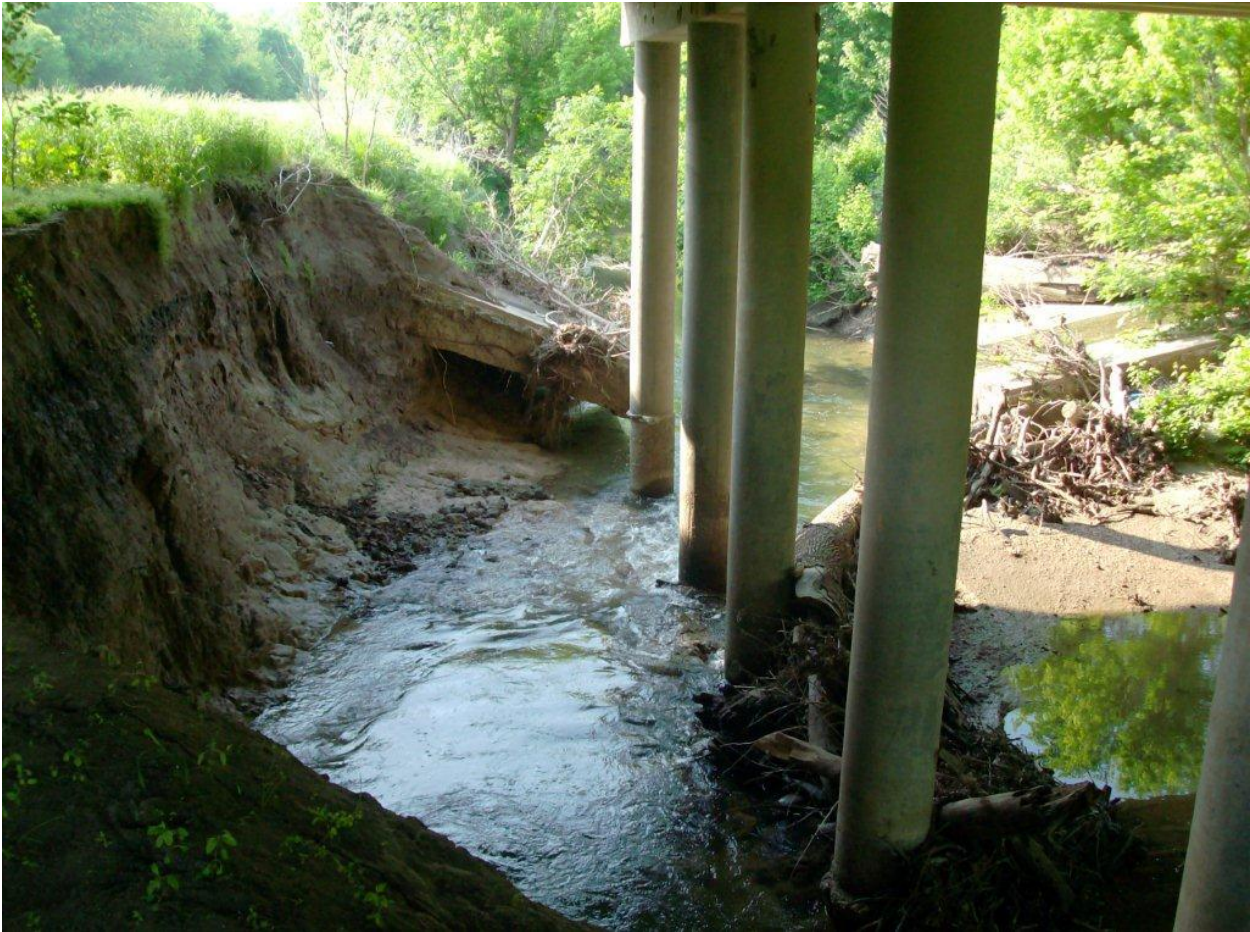
Virginia Parkway bridge over Wilson Creek
