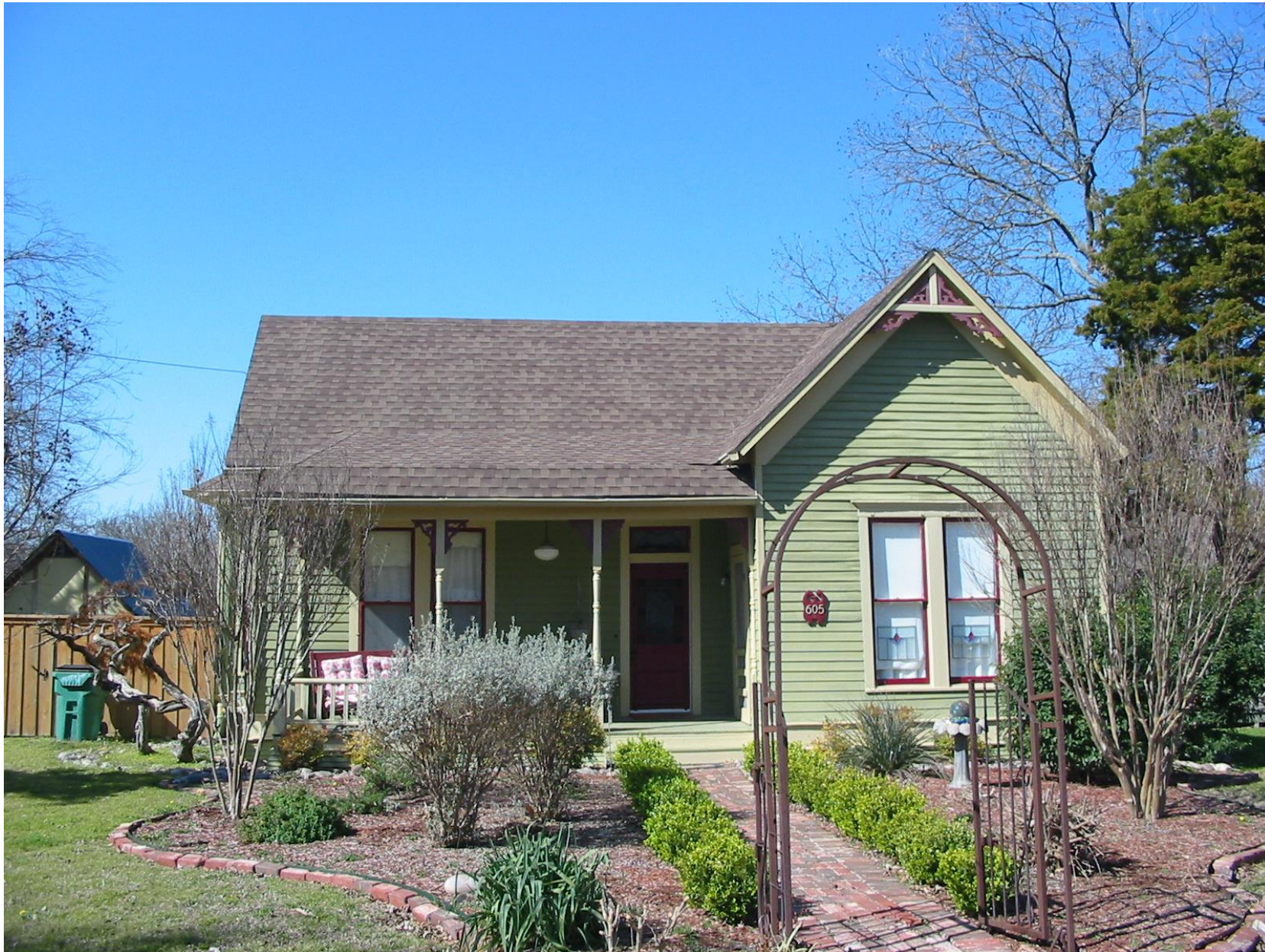
605 N. Bradley Front View 2016
