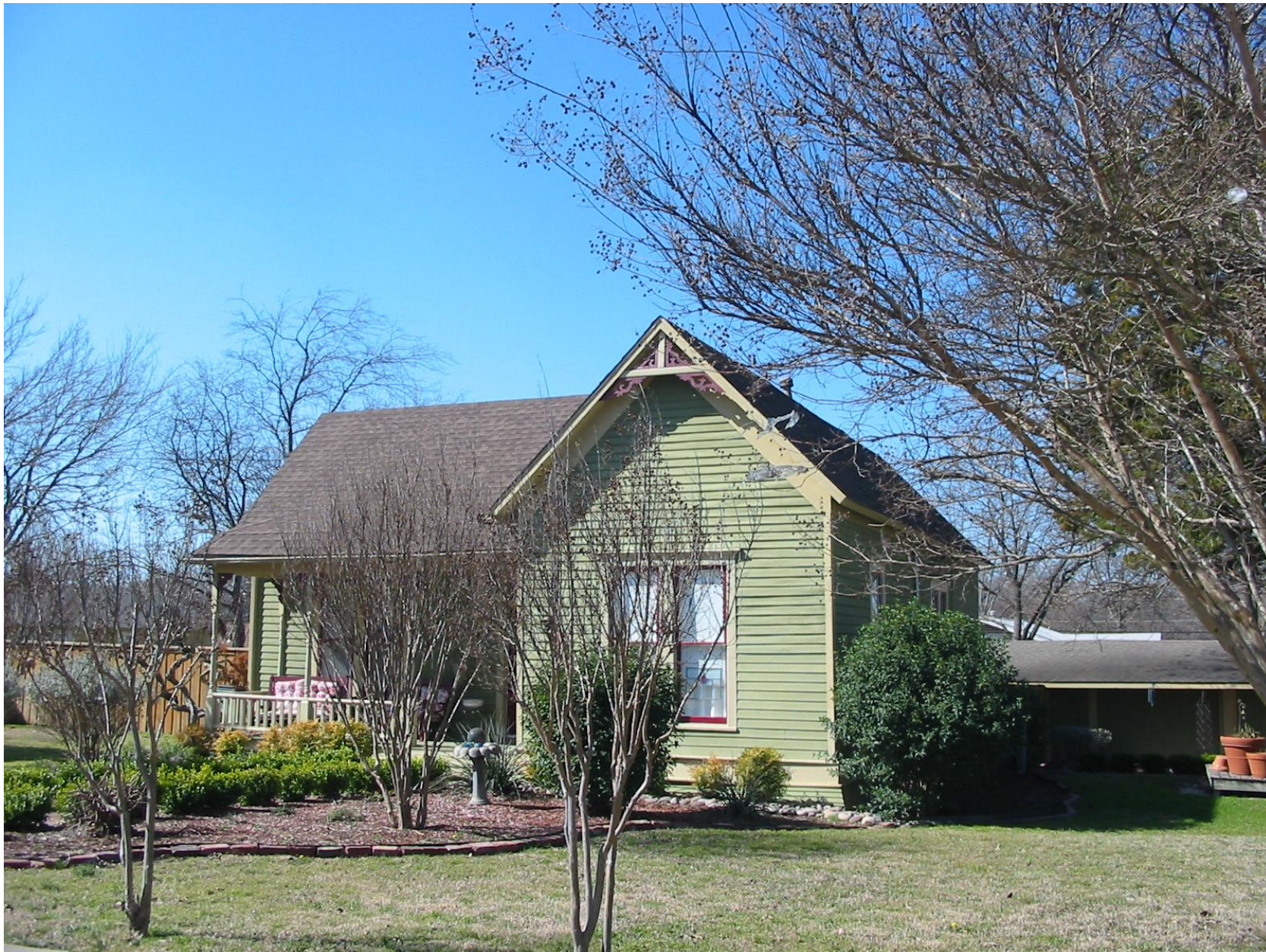
605 N. Bradley Front View 2016
