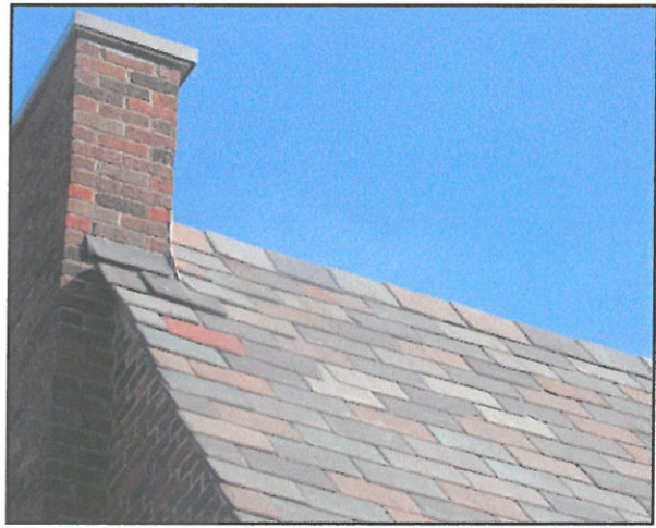
The slate roof is original.
