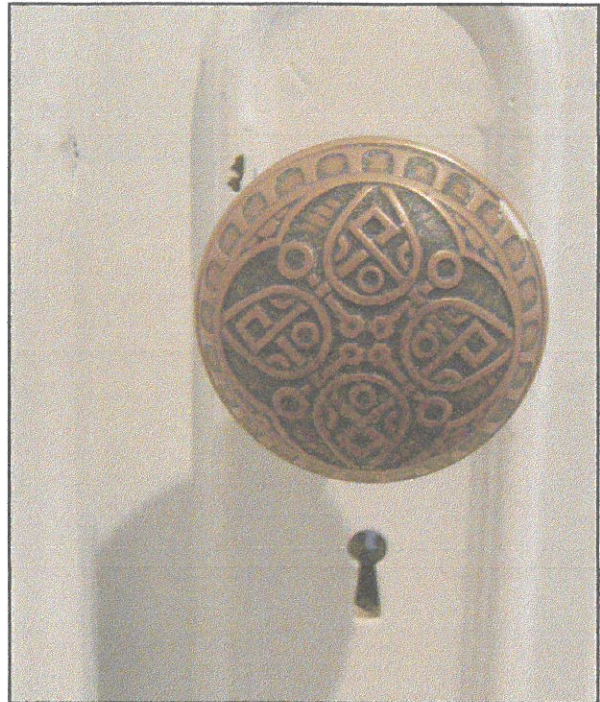
The original door knob remains on an interior door.
