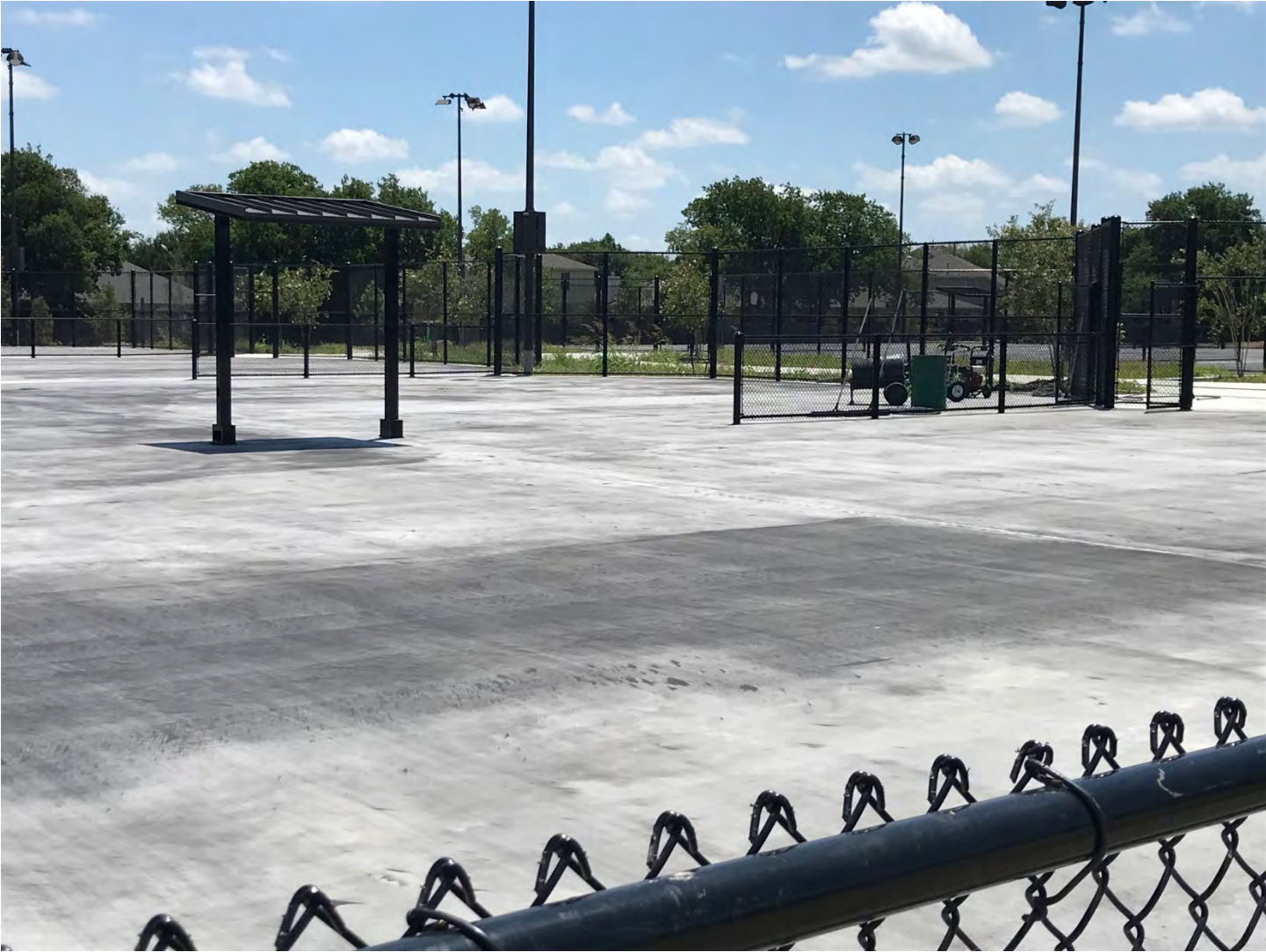
COURTS OF MCKINNEY EXPANSION – OPENING 2019
