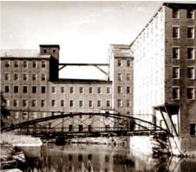
Windows are frequently important visual focal points, especially on simple facades such as this mill building. Replacement of the multi-pane windows with larger panes could dramatically alter the appearance of the building. Photo: NPS files.
