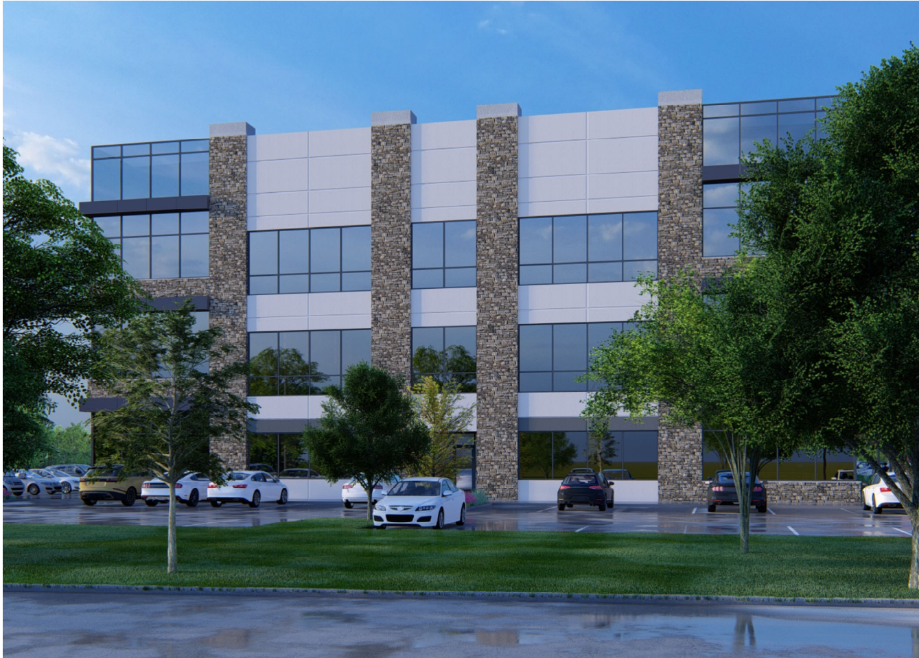
RPM x Construction Office Building East view from Meyer Way
