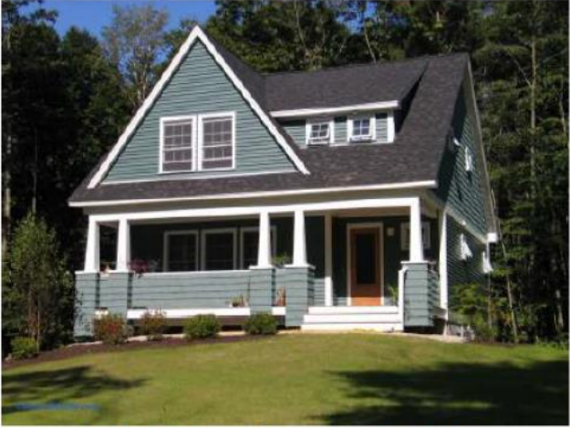
Colonial Revival Twist Style Architectural Example
