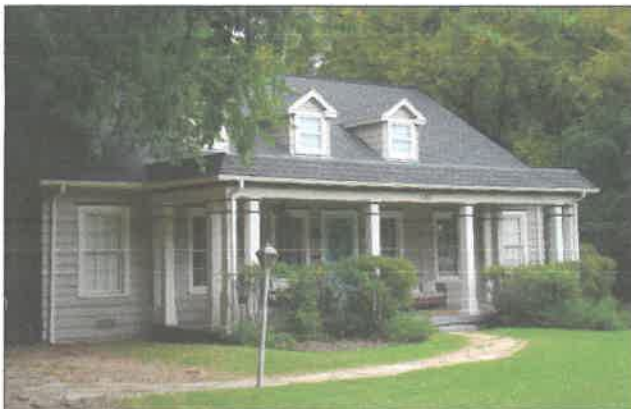
1102 West Virginia Street
