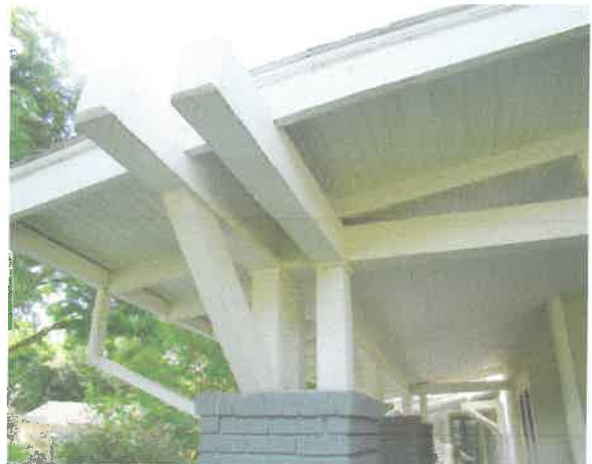
Columns, rafters, and bracing exposed
