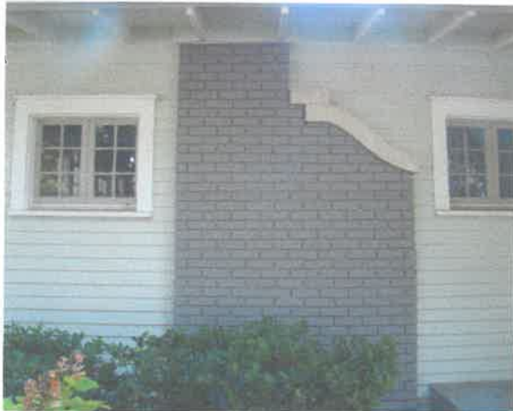
Curved limestone cap on brick
