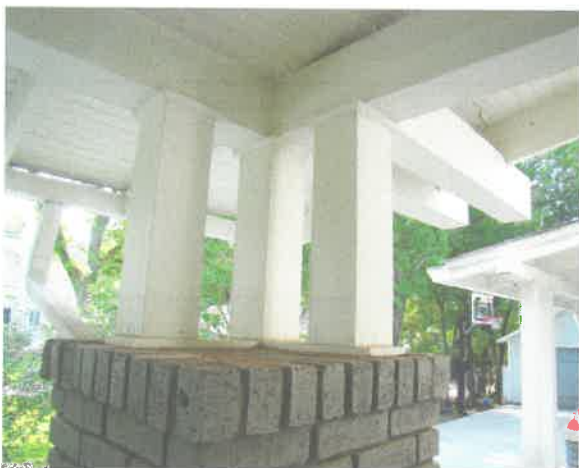
Square, wooden columns on a brick pier
