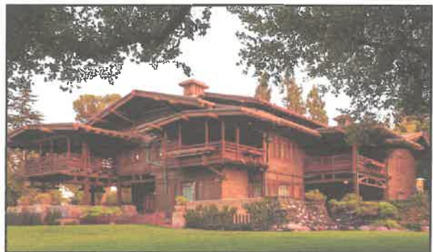
The Gamble House, built in 1908 by Greene & Greene, is considered to be a masterpiece of Arts & Crafts architecture. The Arts & Craft Movement was as much of a labor movement as it was an art movement. It sought better working conditions for laborers. It also sought to recognize the contribution that skilled craftsmen make to creating a more beautiful living environment.
