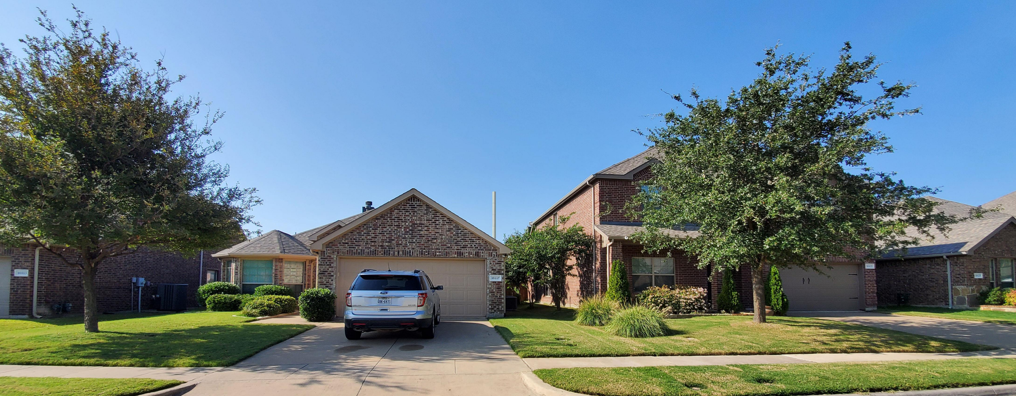
SITE NAME: VERIZON/WESTRIDGE SITE NO. 1640 80' HIGH MONPOLE WITH 3 CANISTERS FURR ELEMENTARY SCHOOL - 551 S. BLUESTEM DR., MCKINNEY, TX 75072
