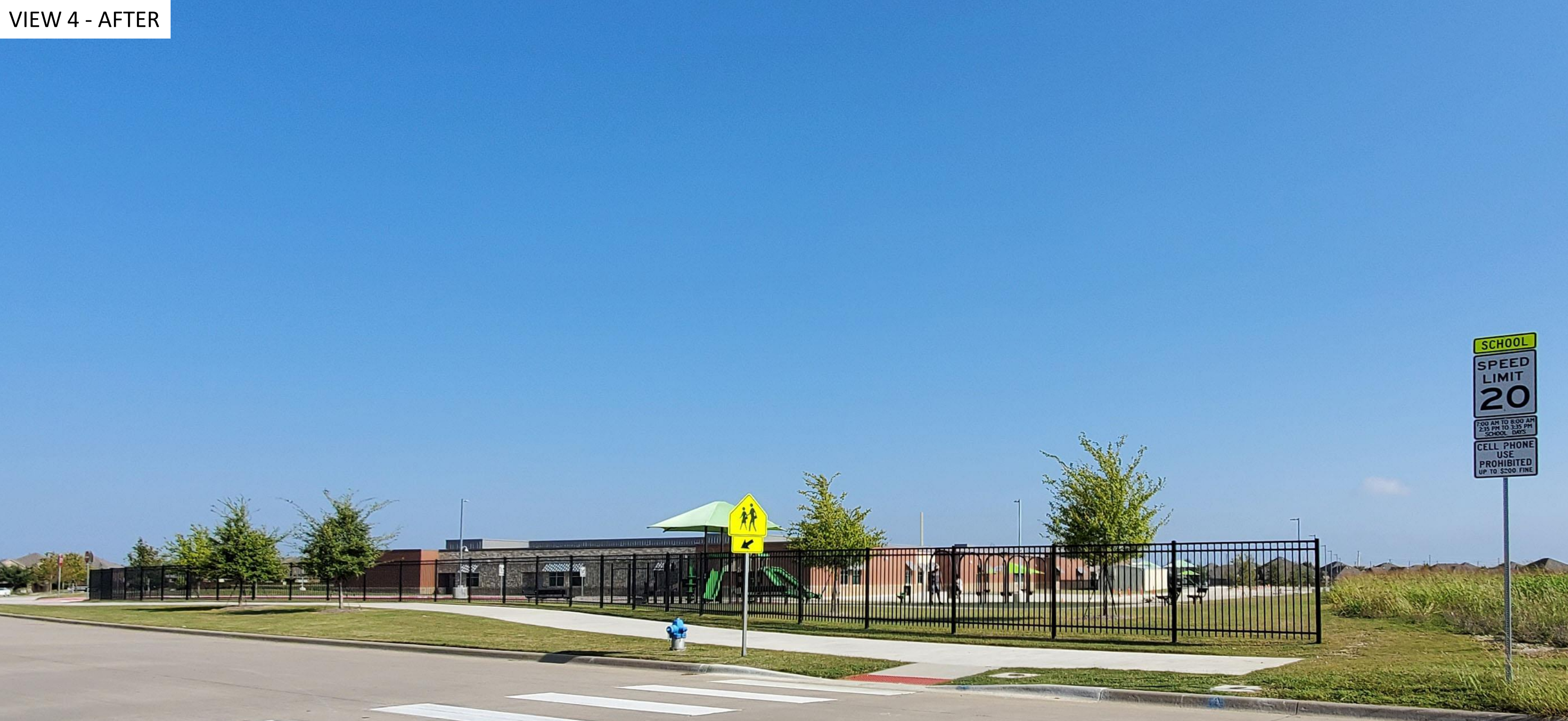
SITE NAME: VERIZON/WESTRIDGE SITE NO. 1640 80' HIGH MONPOLE WITH 3 CANISTERS FURR ELEMENTARY SCHOOL - 551 S. BLUESTEM DR., MCKINNEY, TX 75072
