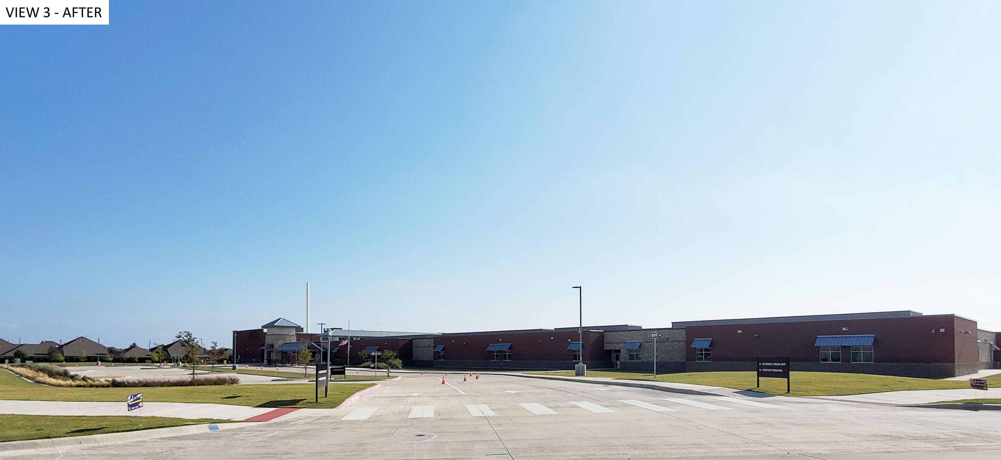
SITE NAME: VERIZON/WESTRIDGE SITE NO. 1640 80' HIGH MONPOLE WITH 3 CANISTERS FURR ELEMENTARY SCHOOL - 551 S. BLUESTEM DR., MCKINNEY, TX 75072
