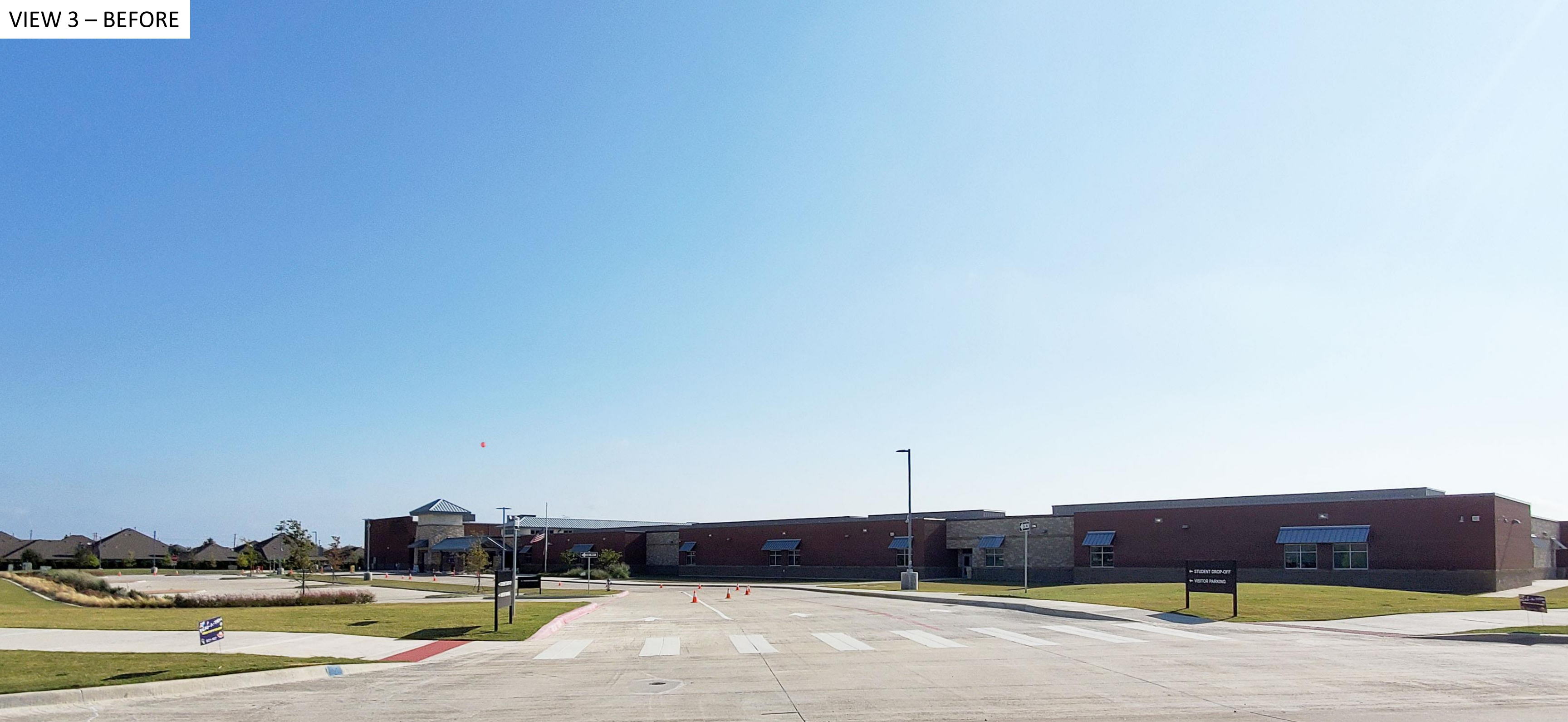
SITE NAME: VERIZON/WESTRIDGE SITE NO. 1640 80' HIGH MONPOLE WITH 3 CANISTERS FURR ELEMENTARY SCHOOL - 551 S. BLUESTEM DR., MCKINNEY, TX 75072
