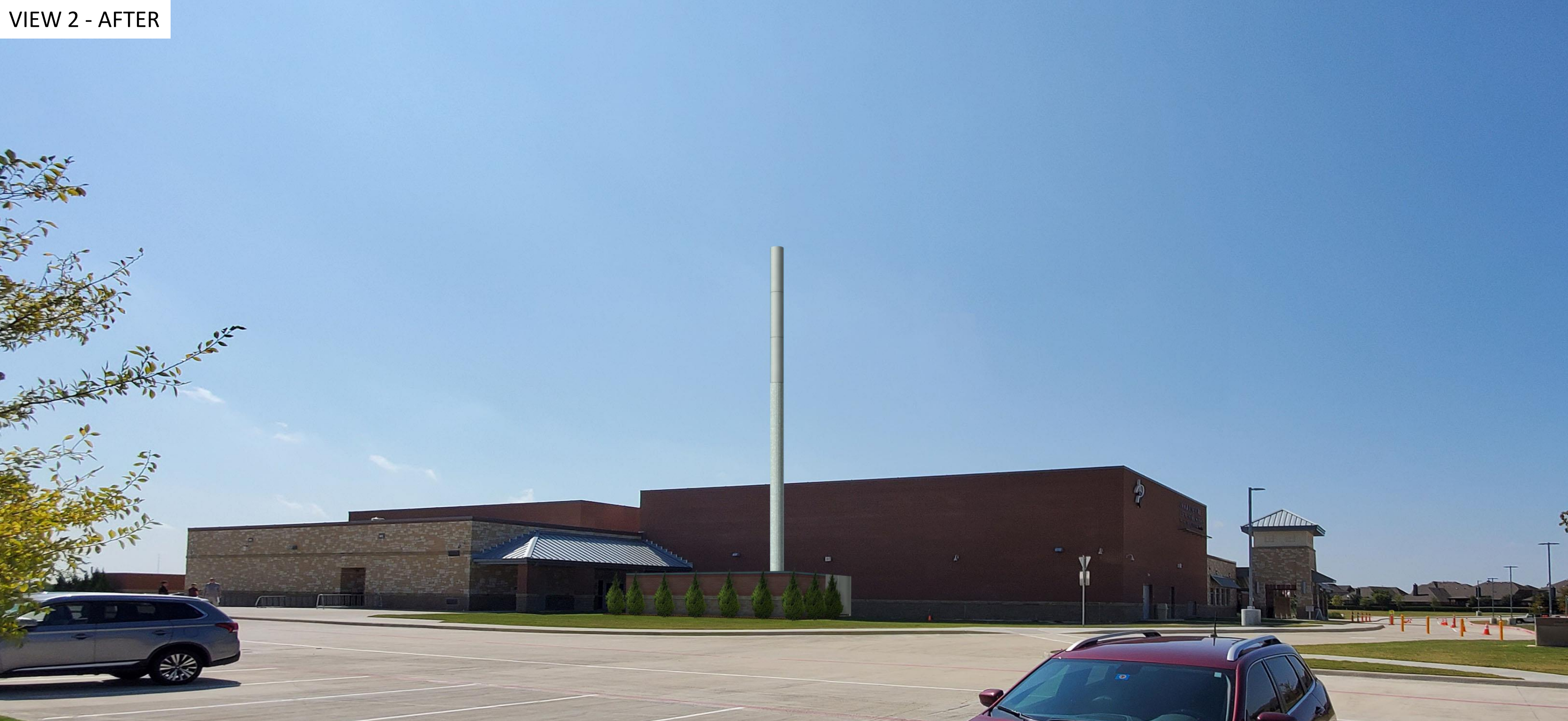
SITE NAME: VERIZON/WESTRIDGE SITE NO. 1640 80' HIGH MONPOLE WITH 3 CANISTERS FURR ELEMENTARY SCHOOL - 551 S. BLUESTEM DR., MCKINNEY, TX 75072
