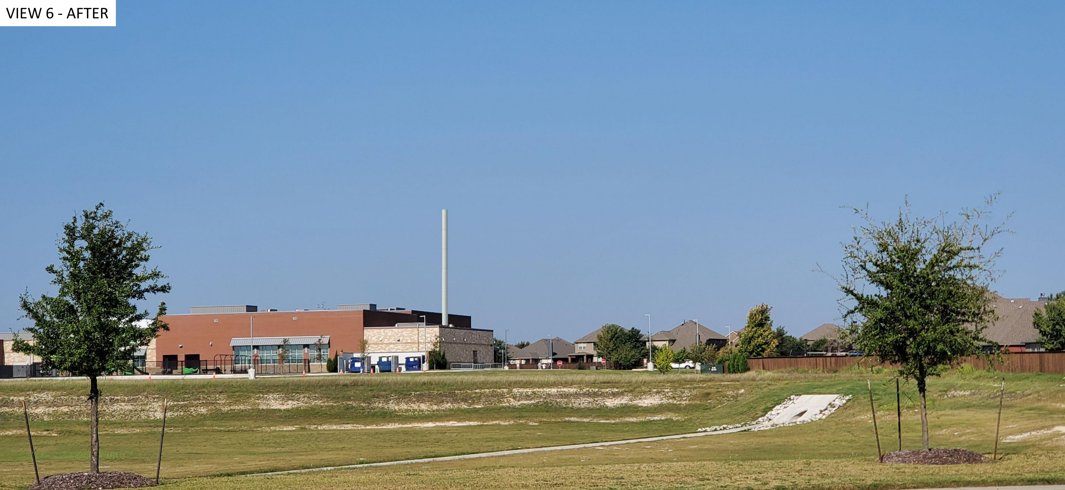
SITE NAME: VERIZON/WESTRIDGE SITE NO. 1640 80' HIGH MONPOLE WITH 3 CANISTERS FURR ELEMENTARY SCHOOL - 551 S. BLUESTEM DR., MCKINNEY, TX 75072
