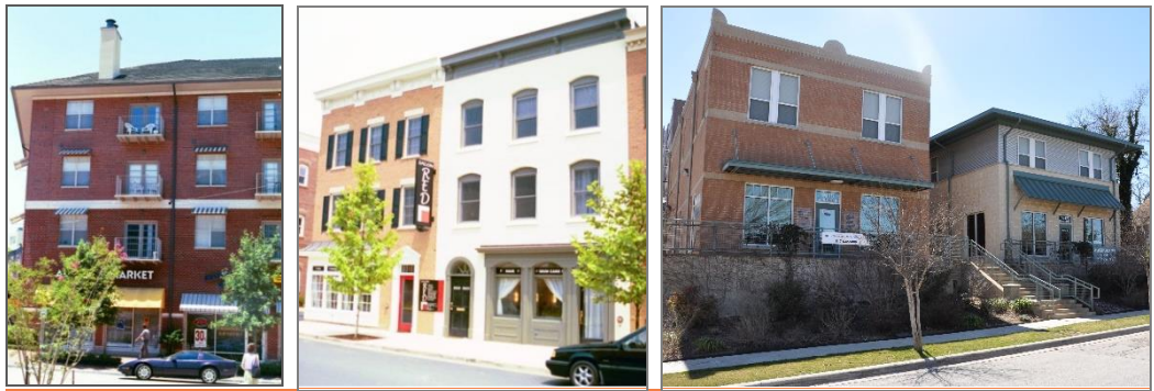
Images showing appropriate window and door designs and proportions for commercial and mixed use buildings.
