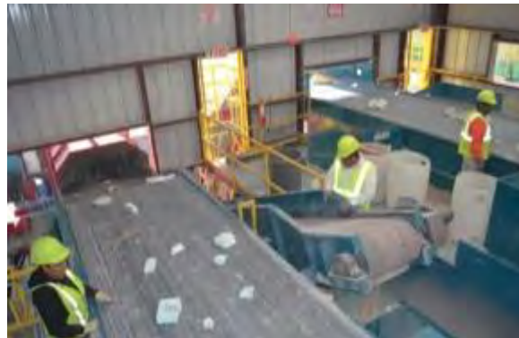
Figure 4-11: Construction MRF Materials Processing Line
