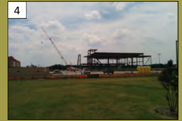
4 Life Fellowship Church 6400 Henneman Way Valuation: $4.7 million Permit Issuance: February 2016
