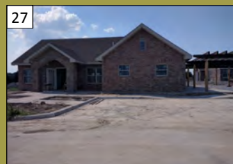
Emerald Cottages 2551 Alma Rd. Valuation: $3.6 million Permit Issuance: November 2014
