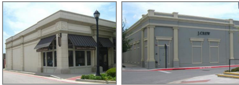
Images showing the side and rear facades buildings finished to match the color and materials of the front facades
