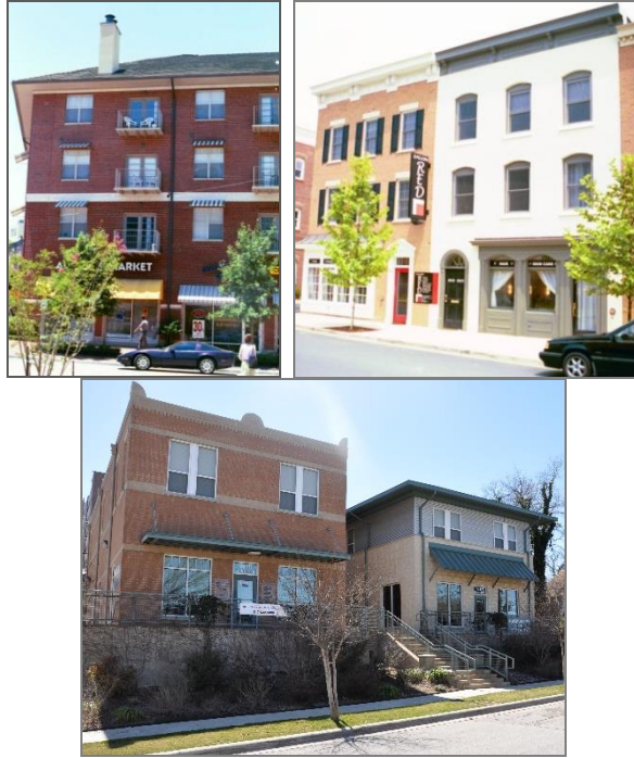
Images showing appropriate window and door designs and proportions for commercial and mixed use buildings.
