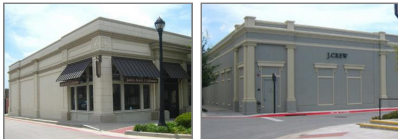
Images showing the side and rear facades buildings finished to match the color and materials of the front facades
