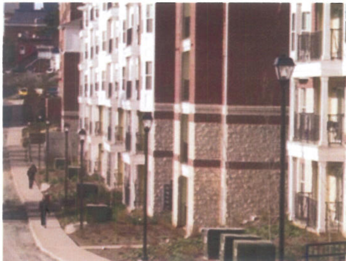
Brick over split-face concrete masonry application.
