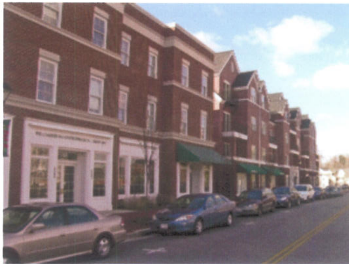
Classically detailed masonry façade with cement fiber board architectural detail.
