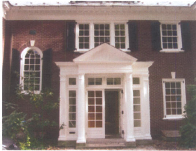
Classical brick façade with fiber-cement panel material. Note the entry gable design similar to the proposed project.
