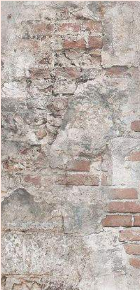
PLASTER LAYERING ON BRICK
