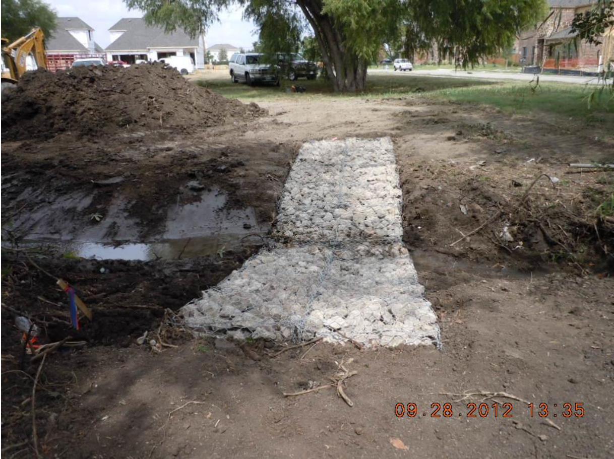
Grade control at a small creek in Village Park
