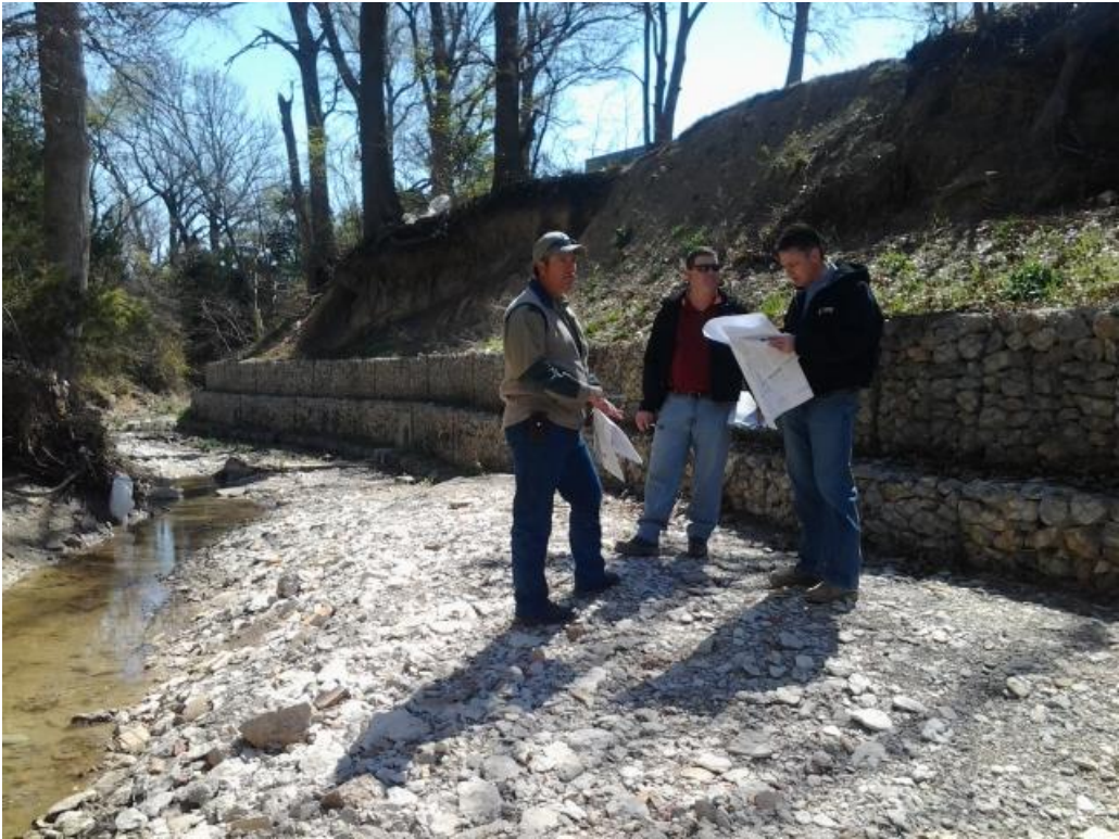
Powerhouse Creek gabion improvements to maximize developable area of lot
