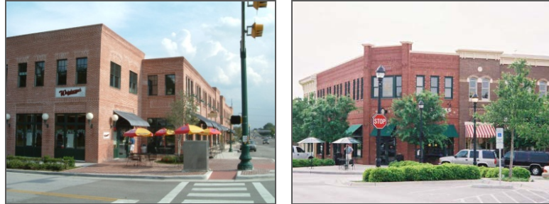
Images showing appropriate building materials within the Historic Core.
