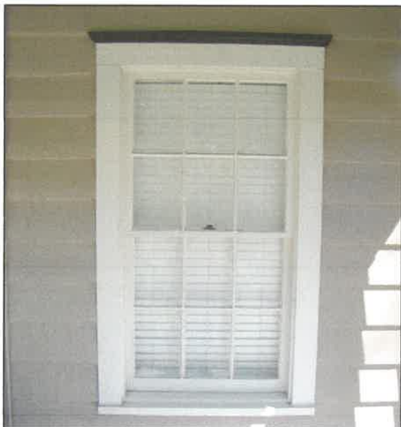
Six-over-six sash windows
